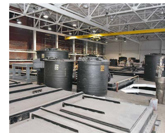
Construction of Nickel Electrolysis Shop-2 (NES-2): technology upgrade and capacity ramp-up
